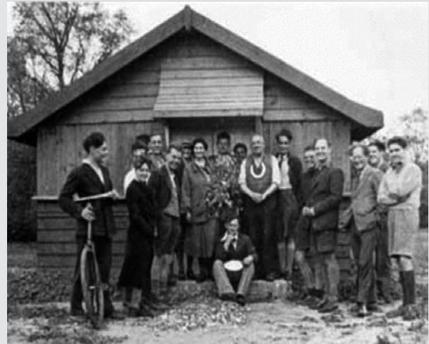
Hawkspur – the first hut built
